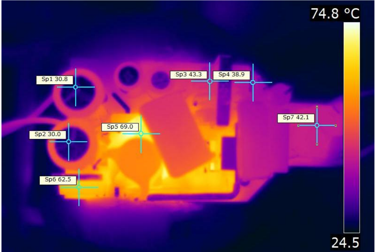
Figure 22 – Open Frame Thermal Scan
