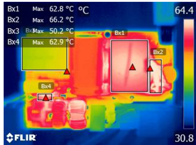
Figure 47 – Top Thermal Image, T_{AMB} = 28.3 °C. Bx1: Transformer Core = 62.8 °C. Bx2: Transformer Wire = 66.2 °C. Bx3: PFC Inductor Core = 50.2 °C. Bx4: Boost Pre-charge Diode = 62.9 °C.
