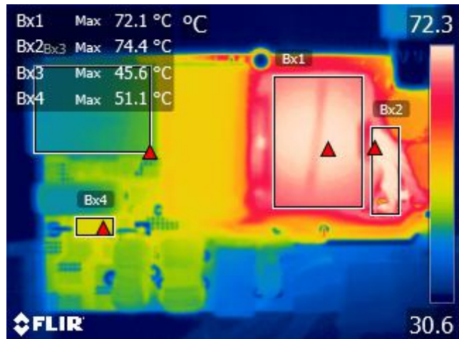
Figure 53 – Top Thermal Image, T_{AMB} = 28.2\text{ °C} . Bx1: Transformer Core = 72.1 °C. Bx2: Transformer Wire = 74.4 °C. Bx3: PFC Inductor Core = 45.6 °C. Bx4: Boost Pre-charge Diode = 51.1 °C.
