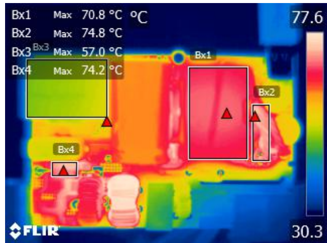
Figure 51 – Top Thermal Image, T_{AMB} = 28.2\text{ °C} . Bx1: Transformer Core = 70.8 °C. Bx2: Transformer Wire = 74.8 °C. Bx3: PFC Inductor Core = 57.0 °C. Bx4: Boost Pre-charge Diode = 74.2 °C.
